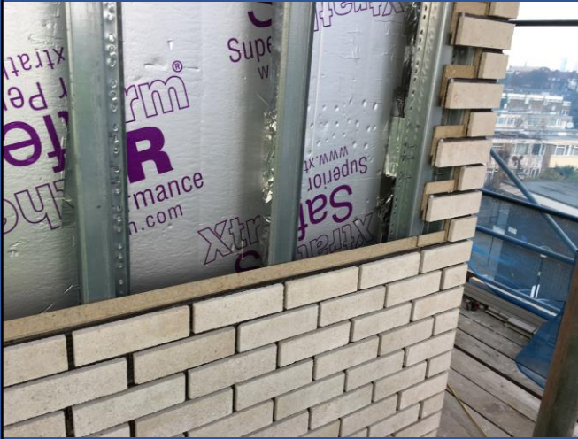
Brick Slip Support and Installation Methods
